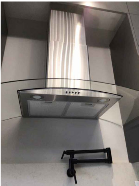
Range/Oven/Cooktop: Exhaust Hood Type Vented
