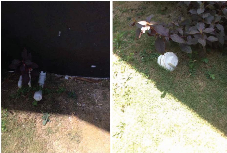
Bathroom Inspection Point
