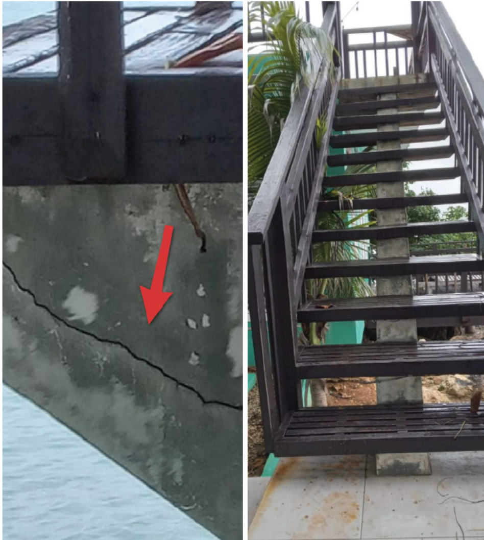
Cottage Deck Staircase
