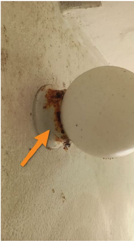
Lights in rooms/exterior
