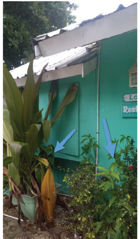
Front of Building
